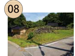
08 Remnants of a Stone Masonry Waterway
