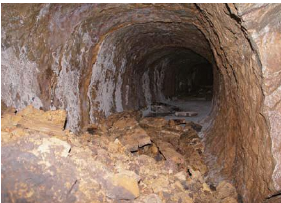
Tunnel mining site (Ogiryama-mabu Tunnel Site, Aikawa area)
